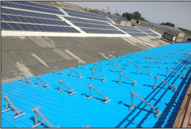
Tin Shed Aluminum Structure
