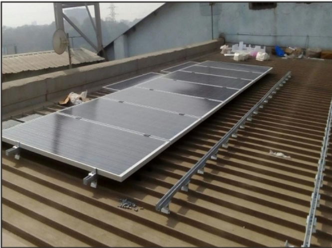
Roof Strut Structure
